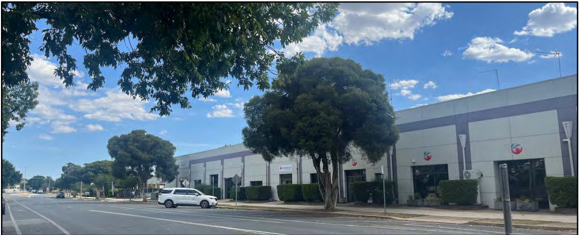
Figure 11: Existing Commercial Buildings – Murray Street (Source: SP 2024)
